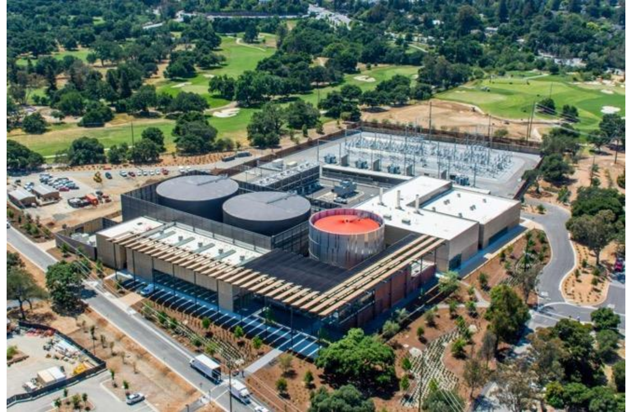
Figure: Stanford's Central Energy Facility, Showing Its Chilled and Hot Water Storage Tanks
